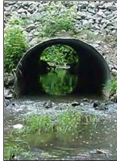
These bottomless or embedded culverts were sized so they are wide enough to carry baseflows without altering stream depth (i.e., width equal to or slightly greater than the average channel width).
