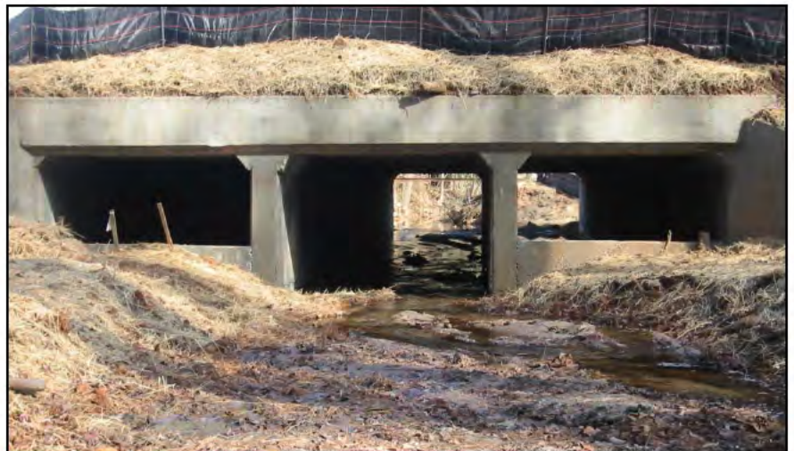
interior and maintain natural flow velocity. Culverts, set at bankfull elevation (top) or with baffles constructed at bankfull height carry flood waters but do not overwiden the channel at baseflow.
