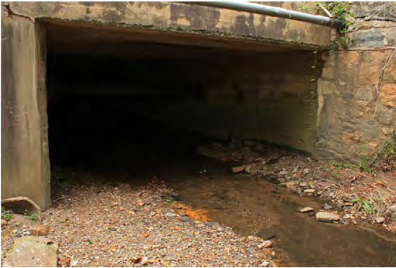
These bottomless or embedded culverts were sized so they are wide enough to carry baseflows without altering stream depth (i.e., width equal to or slightly greater than the average channel width).
